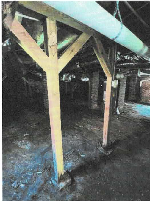
Site Photo 1: “Existing/ original” intermediate joist support.
